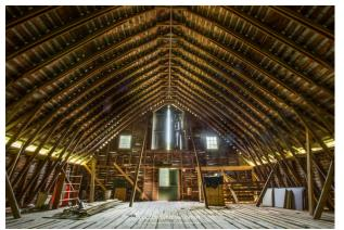
The immense, vaulted loft was used to store hay. The metal track that runs along the length of the loft forms the backbone of the innovative hay-transport system that got the hay up and into the second story of the barn. First, a horse would pull on a rope to hoist a loaded "iron claw" hayfork. Pulleys amplified the pull of the horses and lifted the hay. (The hayfork can be seen on the roof ridge by the visitor stairs. The pulleys are now on display as part of the collection of
